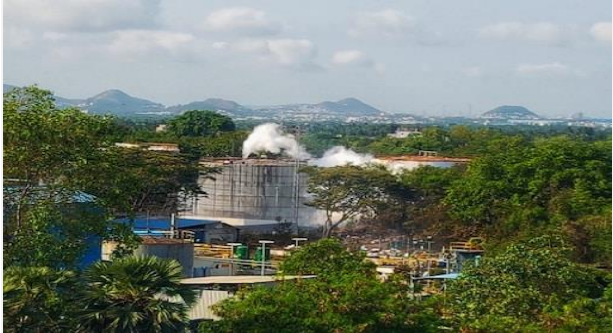
Gas leak in LG Polymers plant in Vizag. (Image: Twitter)
